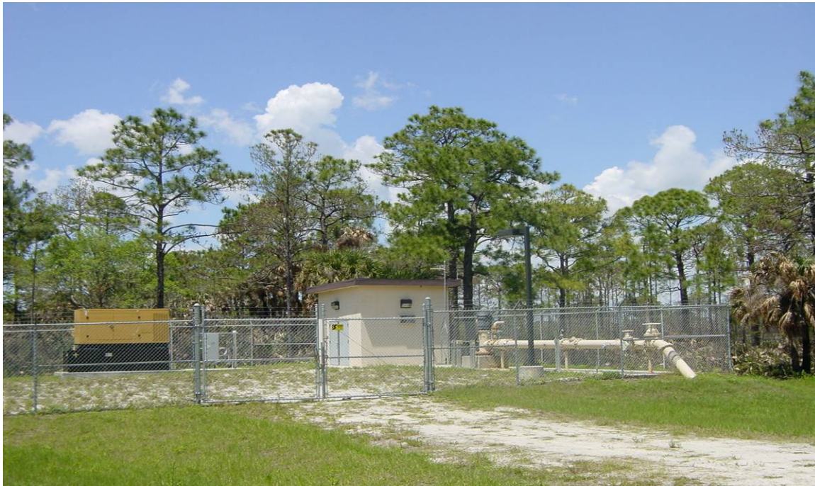
Typical production well site at Carlton Reserve
