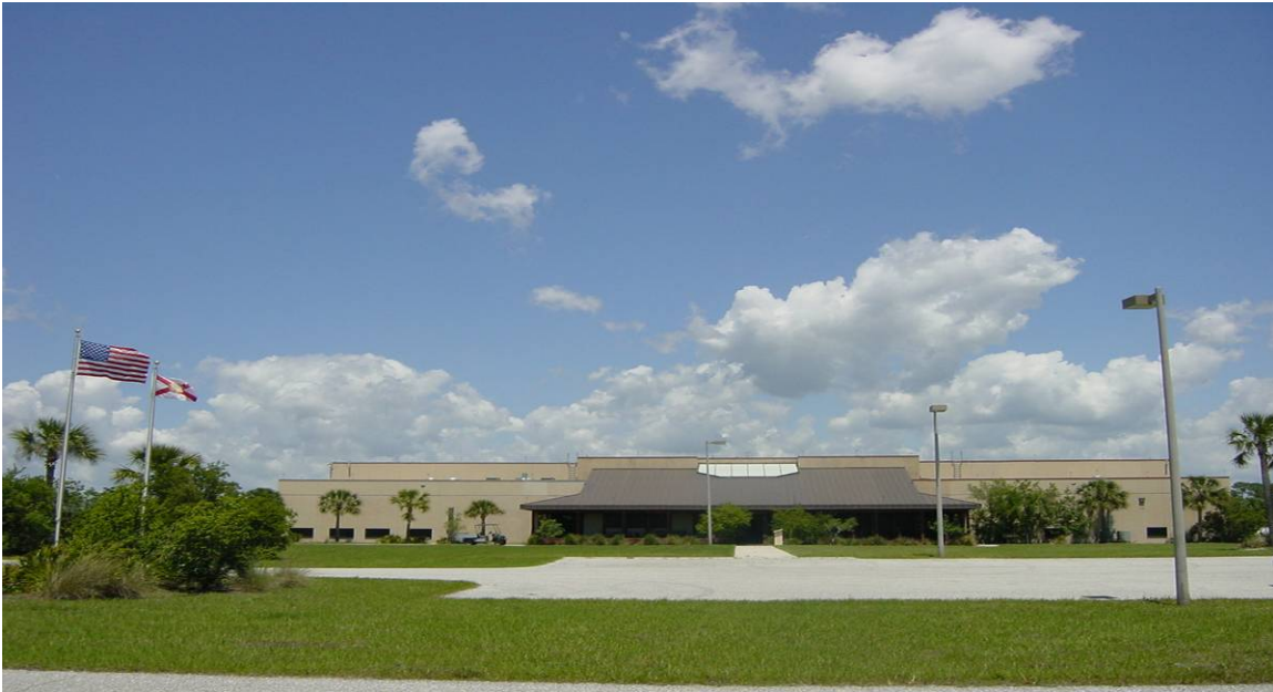
Carlton Water Treatment Facility
